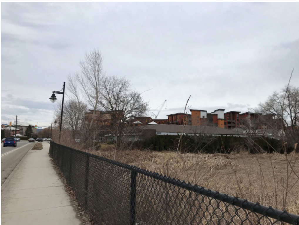
FIG. 18 - Looking north along Lakeshore Rd.
