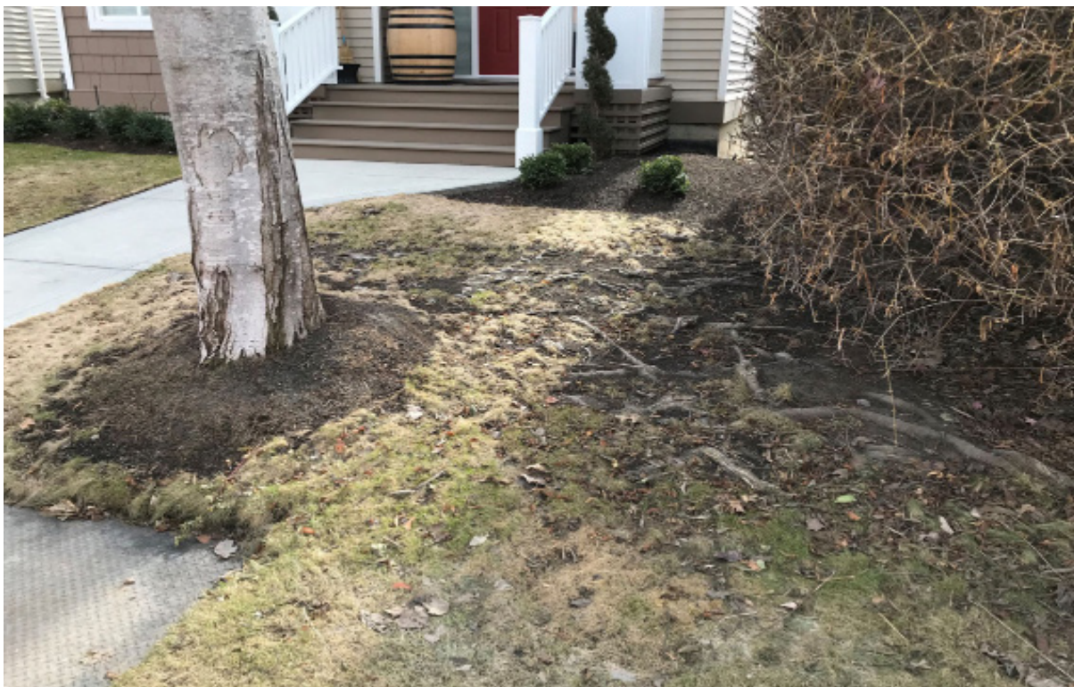
FIG. 16 - Exposed surface roots fo Tree C1 extend into subject property.
